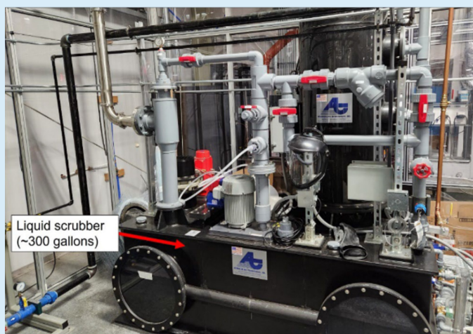
SiC coating system scrubber tank.
